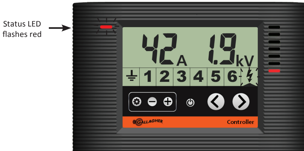
Controller showing the energizer in current alarm
